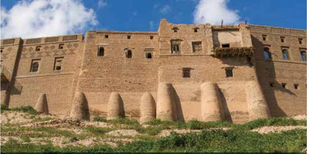
The perimeter walls of Erbil citadel viewed from below the 'tell'. The buttresses give the impression of fortifications, but they support the exterior walls of houses built on the edge of the citadel mound. Photo: Richard Wilding
