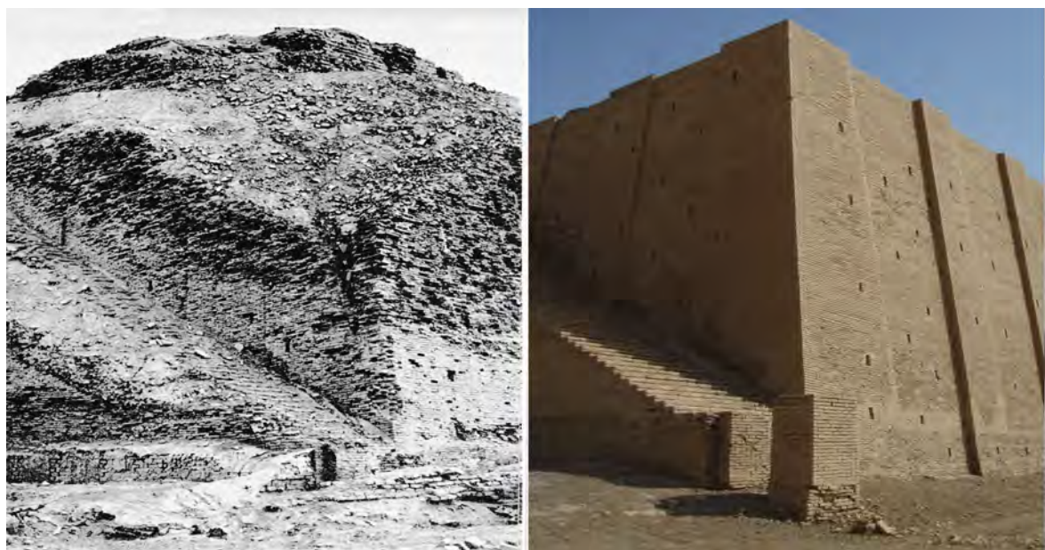
Fig. 7 North corner of the ziggurat, before and after restoration. Photographs cropped. Left: UE5, Pl. 42. Right: Kaufingdude 2007. CC BY-SA 3.0.
