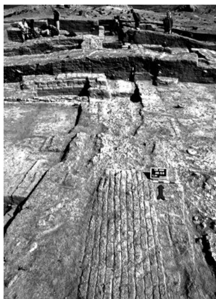
Figure 27: Alley in Area G, from south, with fallen mud-brick in foreground
