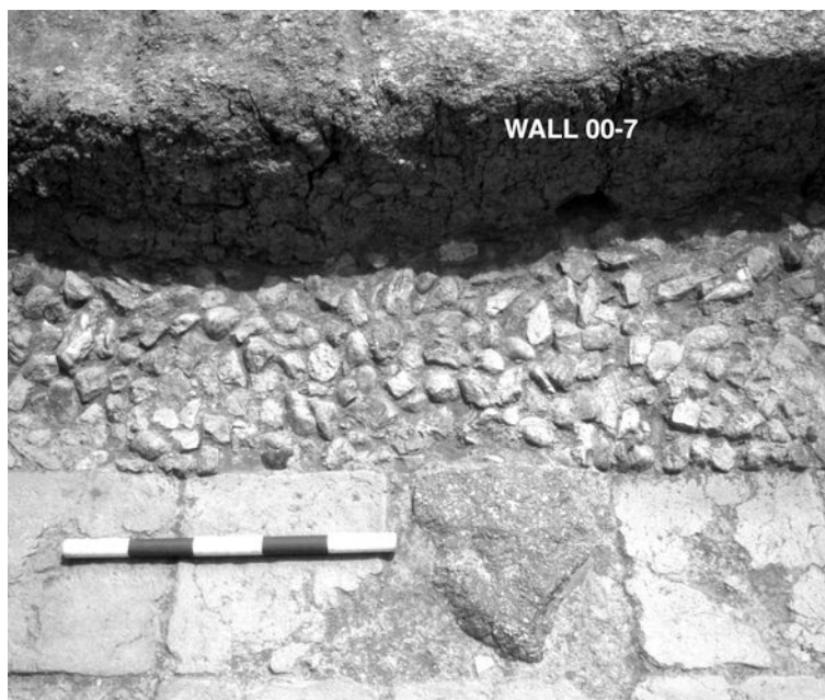
Figure 12: Detail of cobble edging in courtyard of Building III, Area A Phase II, from north
