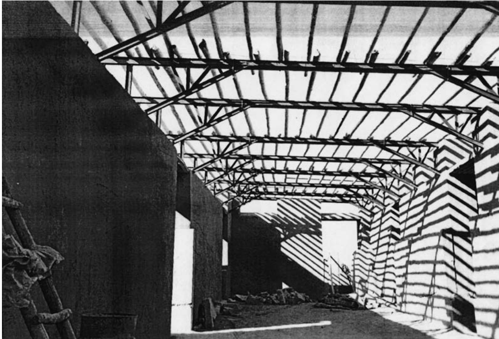
Fig. 6-e. Reconstruction in progress.
