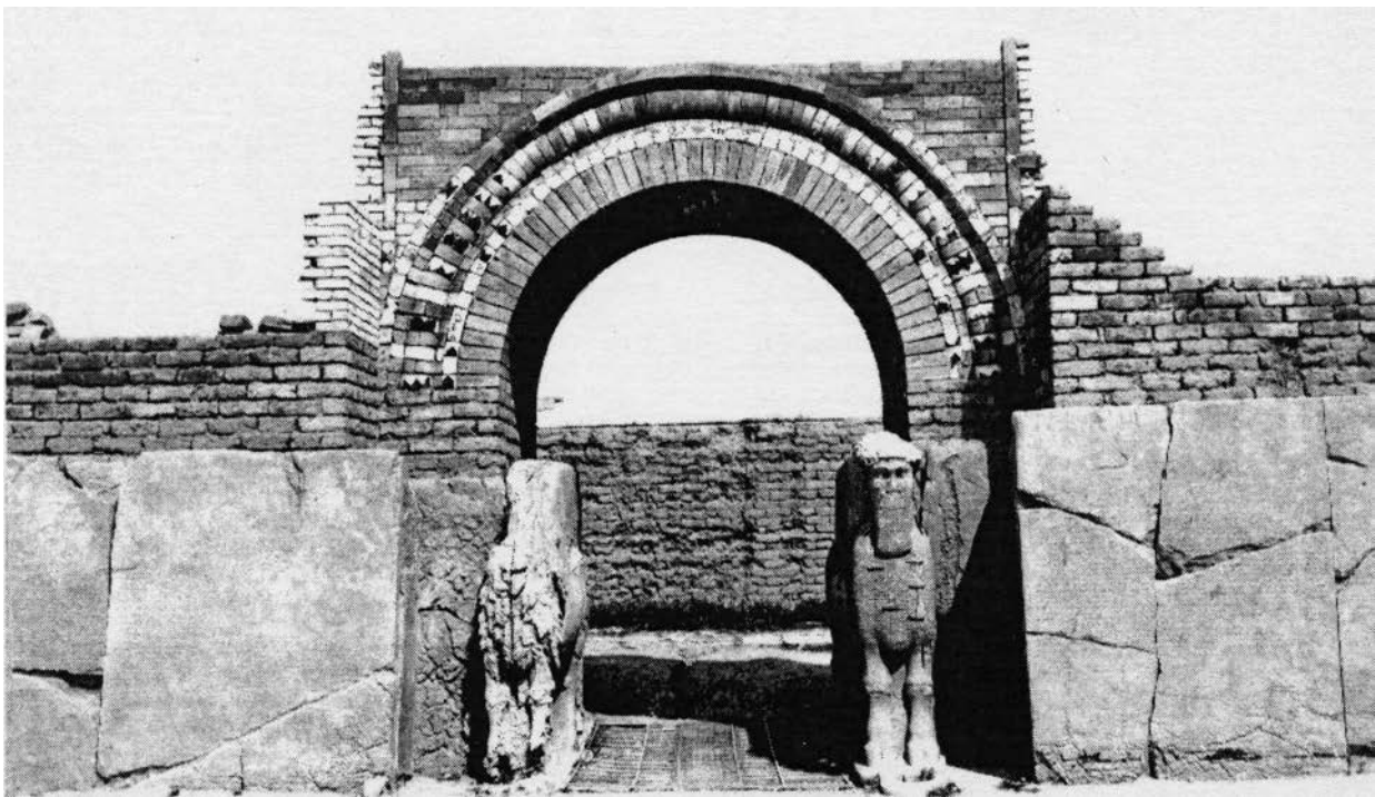
Fig. 6-f. Part of the northern façade of Courtyard Y, entrance F with winged bulls. The arch is of modern construction.
