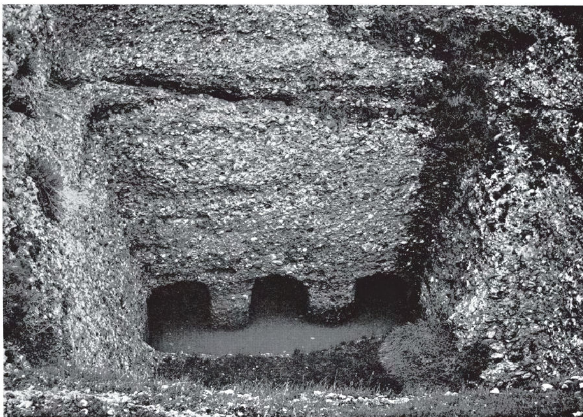
b. Sluice openings in the east shaft of the Negūb tunnel
